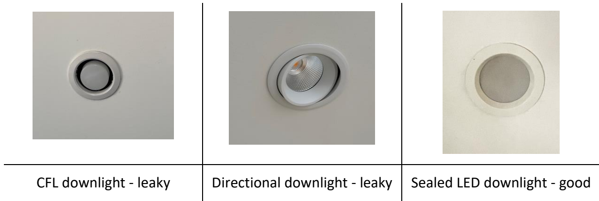
Figure 22 Downlight types
