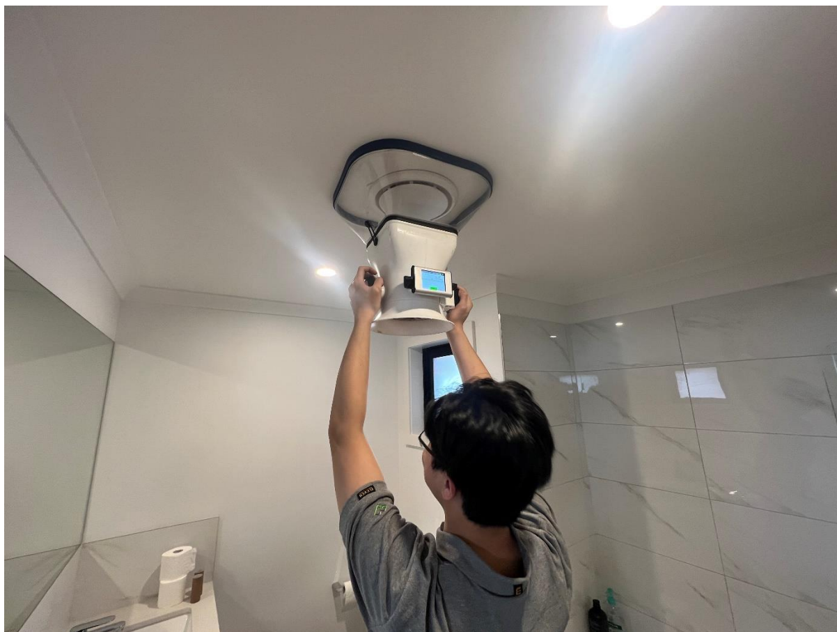
Figure 31 Measuring exhaust fan ventilation
